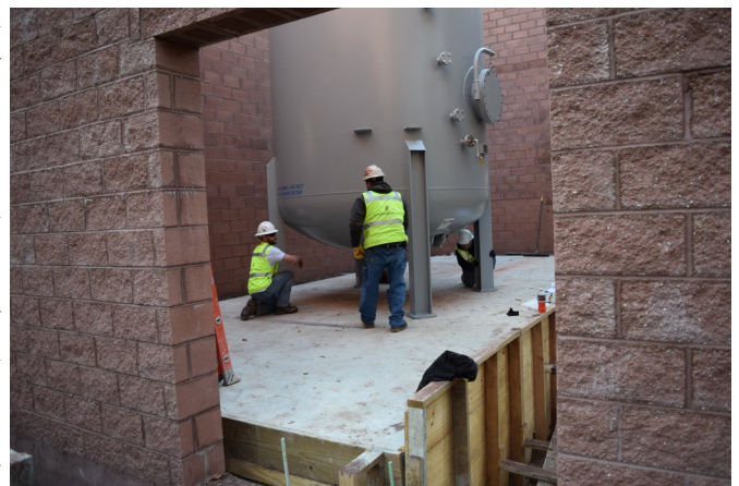
Installation of GAC Unit for one of the HWSA Wells
